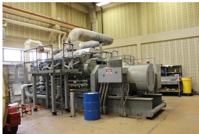
Superior 600 kW Engine. Source Iowa Environmental Council
