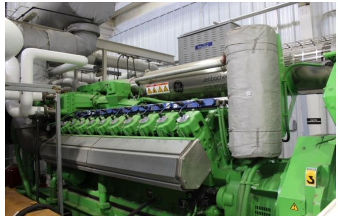
New 1.4 MW Jenbacher Engine. Source: Iowa Environmental Council
