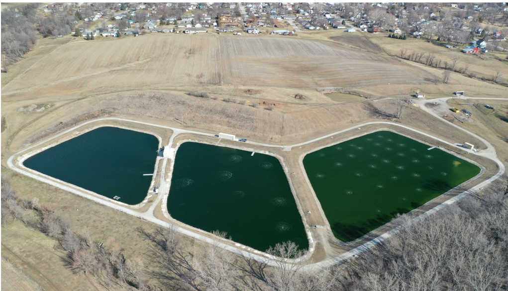
Aerated Continuous Discharge Lagoon
