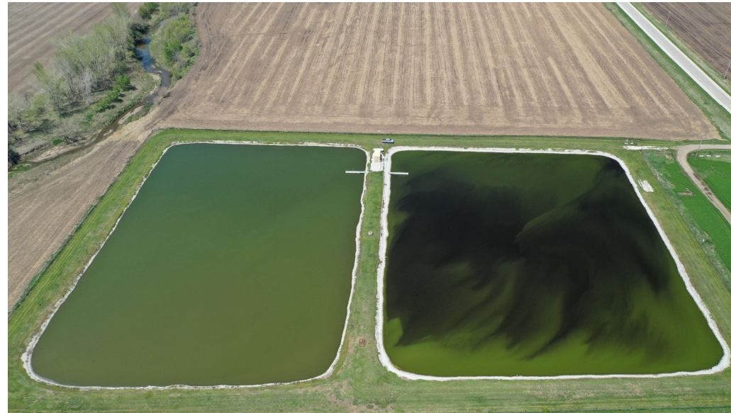
Controlled Discharge Lagoons
