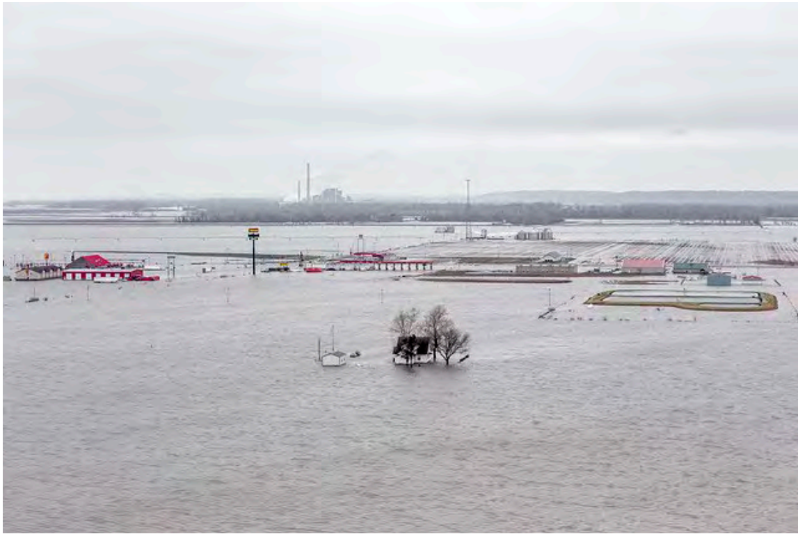
March 28, 2019 – I-29 & US 34 Interchange, Iowa DOT
