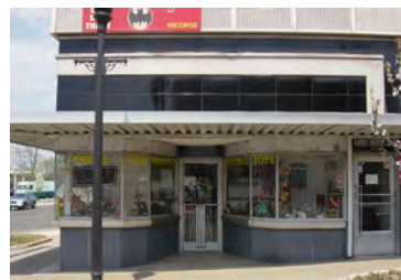
Retractable awnings are ideal since they can be rolled up during the evening to allow radiant cooling during the summer, although fixed ones are suitable. Fixed canopies should be maintained at a shallow slope to allow enough light into the storefront.
