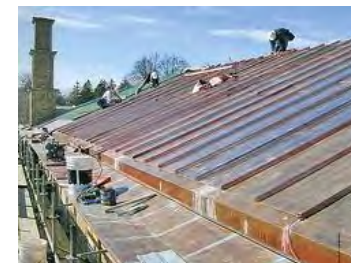
Maintaining original roofing materials, such as standing seam copper (above) should be a priority. If replacement is necessary, metal roofs can be ordered with “cool roof” reflective coatings.
