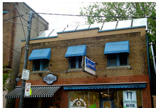
Design guidelines can address where solar panels should be placed on a historic commercial building. In this instance, panels should have been placed to rear where they cannot be seen at street level.
