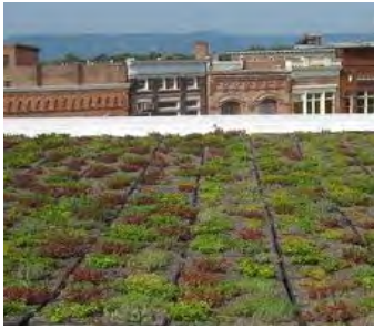
Green roofs can provide energy efficiency savings. Buildings with minimal sloped roofs and adequate parapet walls and structural load capacity can be ideal candidates for green roofs. - photo courtesy of gbNYC
