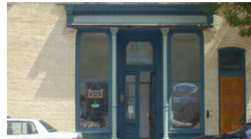
Historic windows and doorways should be kept in good condition and not removed. All doorways and windows should be checked for air infiltration and weatherstripped and sealed accordingly.
