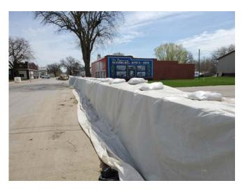
Figure 3.4-7 Flood wall in Hamburg.
