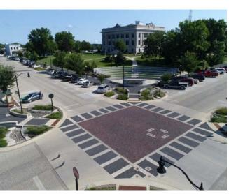
Example of stormwater bumpout intersection
