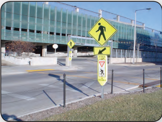
A raised pedestrian crosswalk on the University of Iowa campus.
